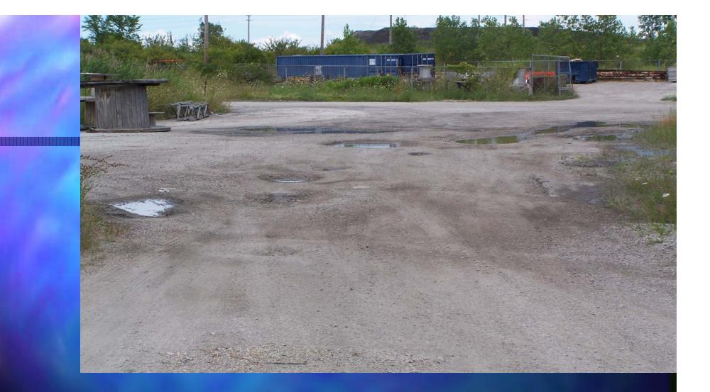
POTHOLES AND RUTS RETAIN WATER AND ARE SLIPPING HAZARDS IN THE WINTER...... THEY ARE HARD ON VEHICLES, OPERATORS AND PASSENGERS.
